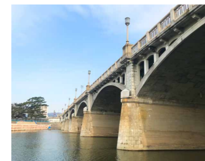
Muko Ohashi Bridge
